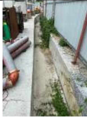
Fig 3: Existing 1m (W) x 1m (H) in the site
