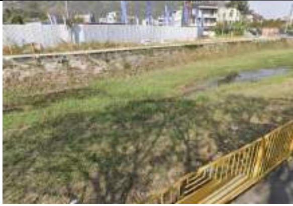
Fig 2b: Final Discharge to Wong Tong Stream ( Maintained by DSD)
