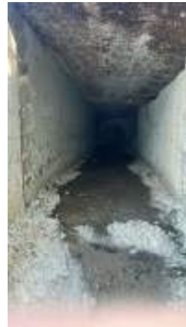
Fig 5 Existing Underground 1000mm box culvet
