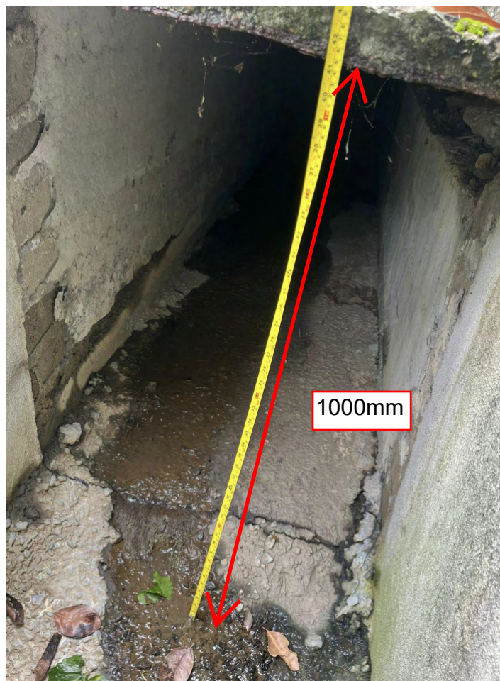
Dimension of 1000mm Box Culvert
