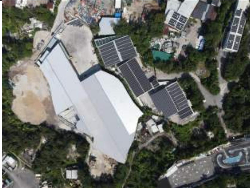
Aerial Photo: Overview of the Site
