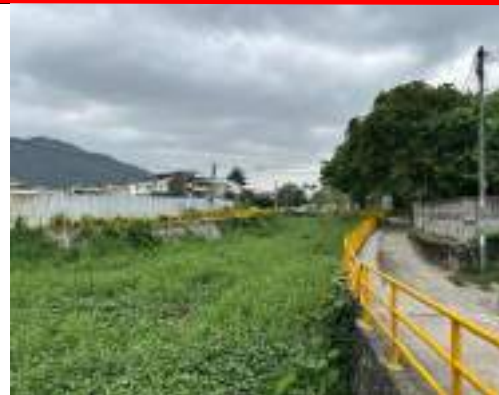
Fig 2a: Final Discharge to Wong Tong Stream ( Maintained by DSD)
