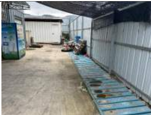
Fig 4: Existing 1m (W) x 1m (H) in the site
